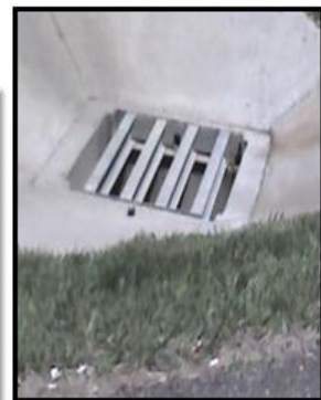
Photograph 8-7. CDOT Type C Grate Inlet (UDFCD Volume 1)
