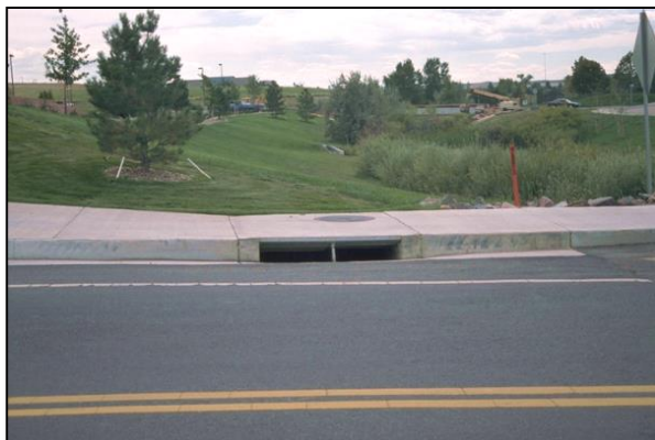
Photograph 8-1. Inlet in sump
