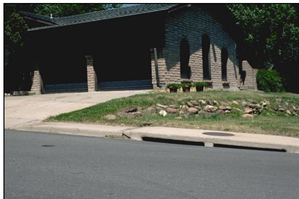
Photograph 8-2. Inlet on grade
