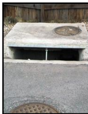
Photograph 8-5. CDOT Type R Curb Opening Inlet (UDFCD Volume 1)
